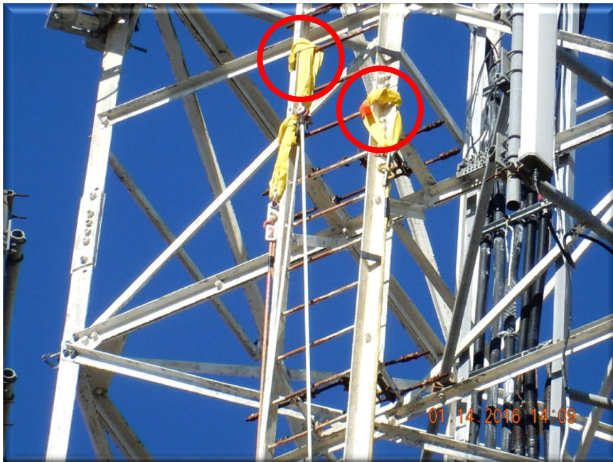
Rigging Attached to Climbing Facility
