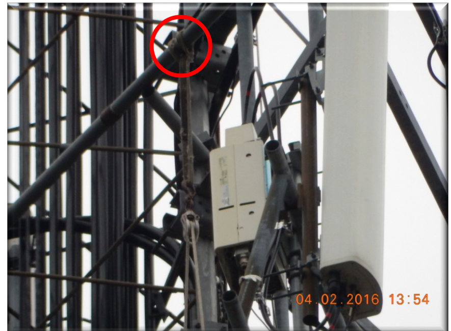
Rigging Attached to Mount Tie-Back
