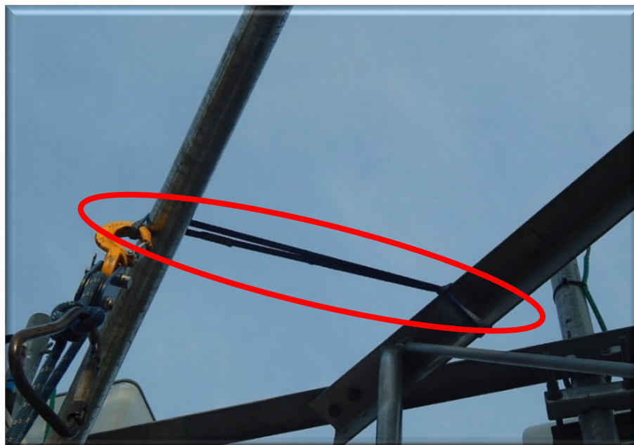
PPE Sling & Attached to Mount Standoff
