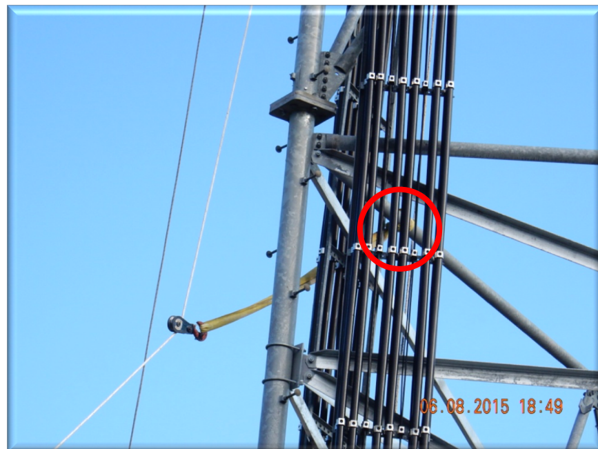
Rigging Attached to Lattice Bracing
